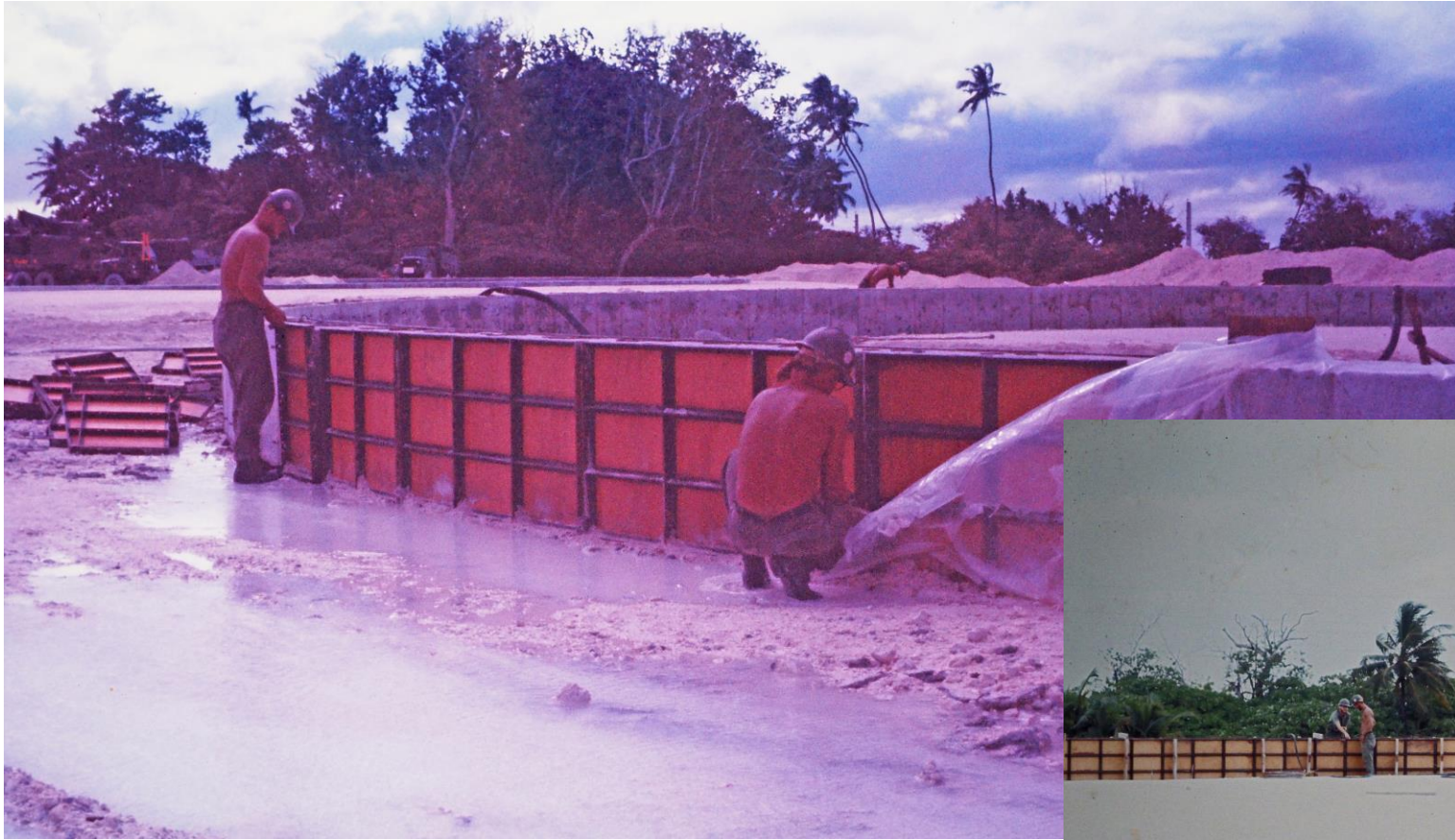
NMCB 62's Seabees built the concrete base pads and the support foundation for each of the tanks in the tank farm.
