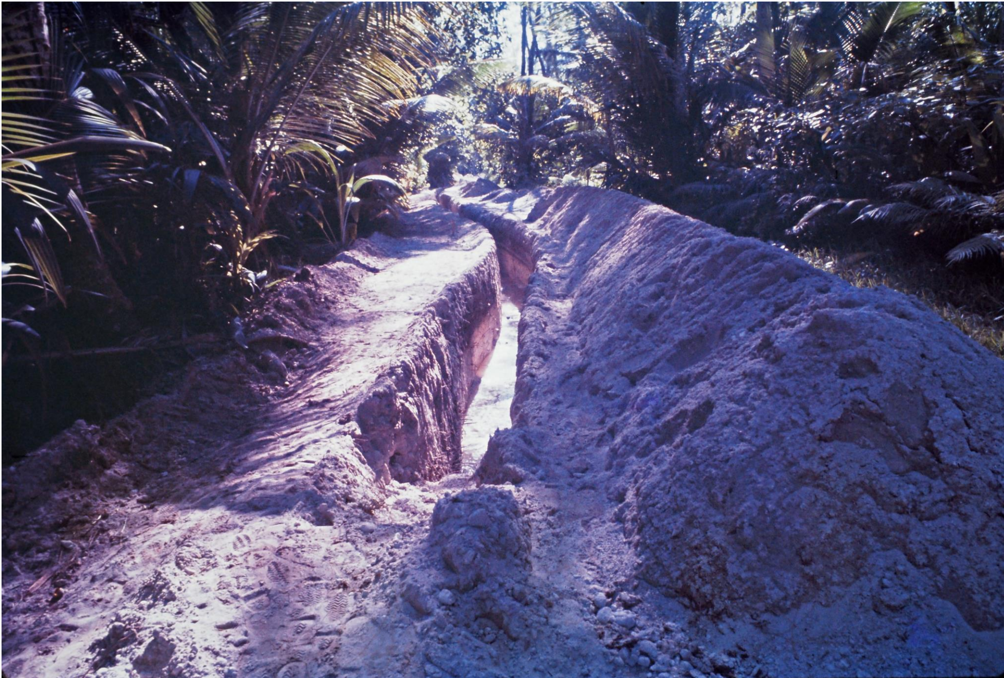
Trench for a segment of the underground piping for the water lines.
