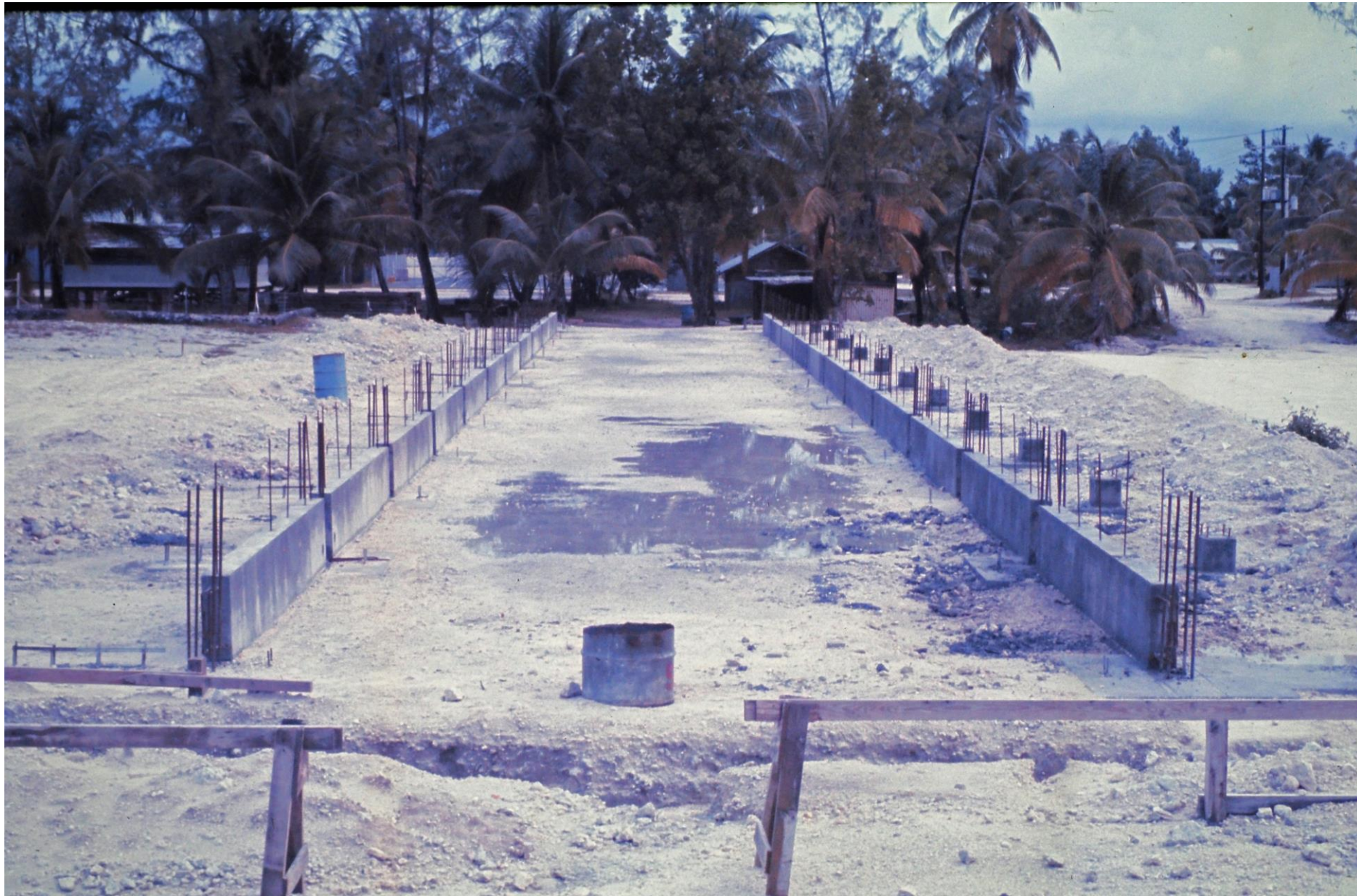
Grade beams and reinforcing steel or “rebar” ready for the structural walls.
